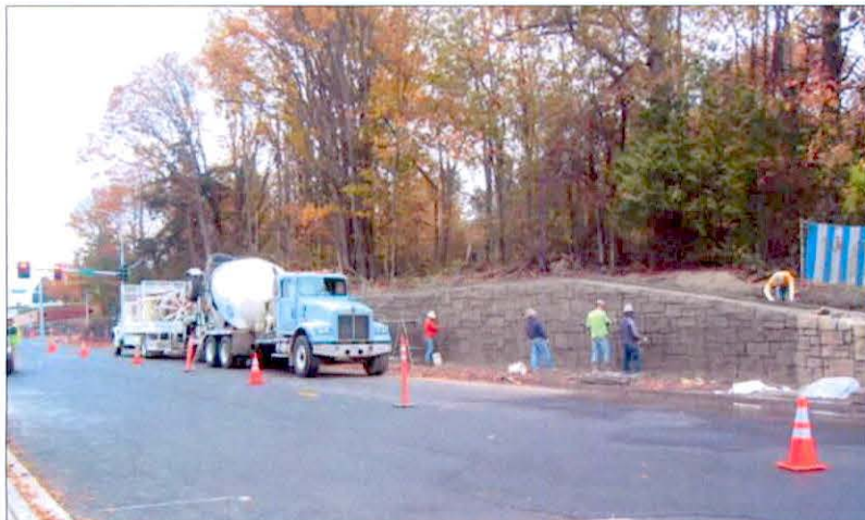
Finishing work on retaining walls along 16th Avenue South.
